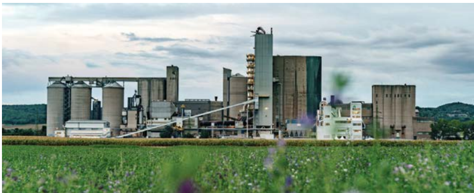
Holcim Werk in Mannersdorf
